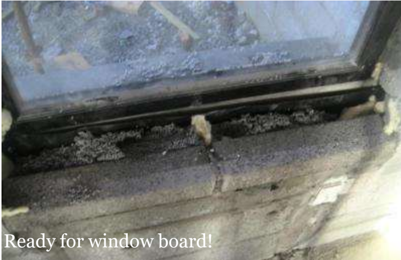
Bay window – gaps to insulation
