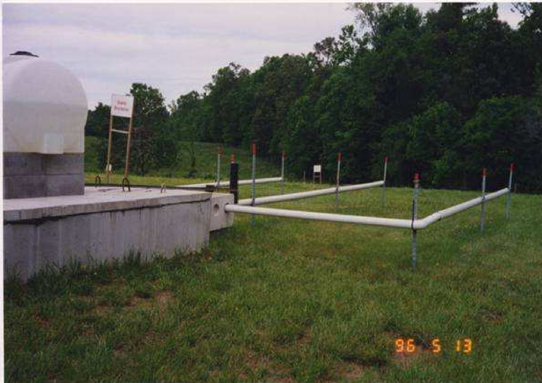
SEPTIC TANK AND DRAIN FIELD
